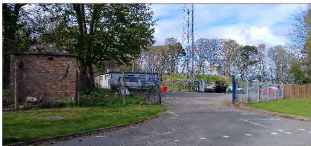
Plate 23: NW facing view of RAF Filter Block (Asset 10)
