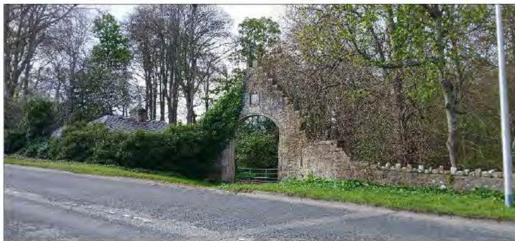
Plate 25: SW facing view of Inshes Archway (Asset 13)
