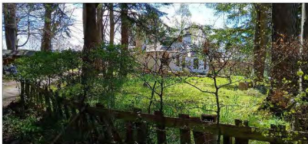
Plate 24: South facing view of Helen's Lodge (Asset 11)
