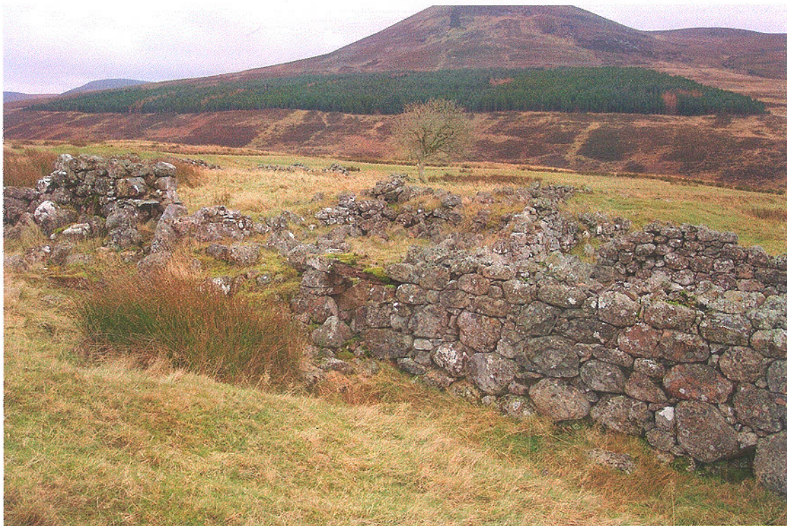
Plate 20. Features 137 & 138. Enclosure (right) and building remains (left) of farmstead of Lower Breac-achadh. Wall with sheep creep (centre) is 0.8m high. GR 284679 911573
