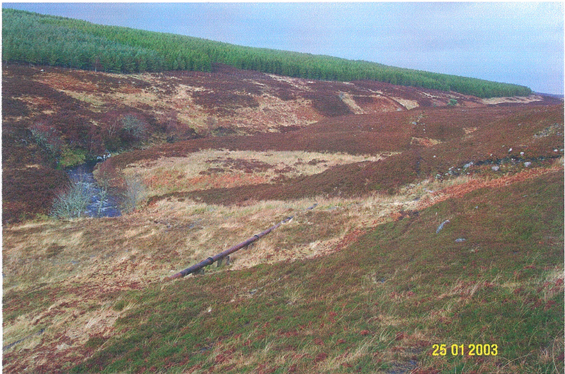
Plate 16. Feature 069. 300mm diameter water pipeline, at this particular location on concrete stilts, formerly carrying water from the dam across Allt a'Mhuilinn to the hydro-electric power generating station of Feature 052. GR 282772 911696
