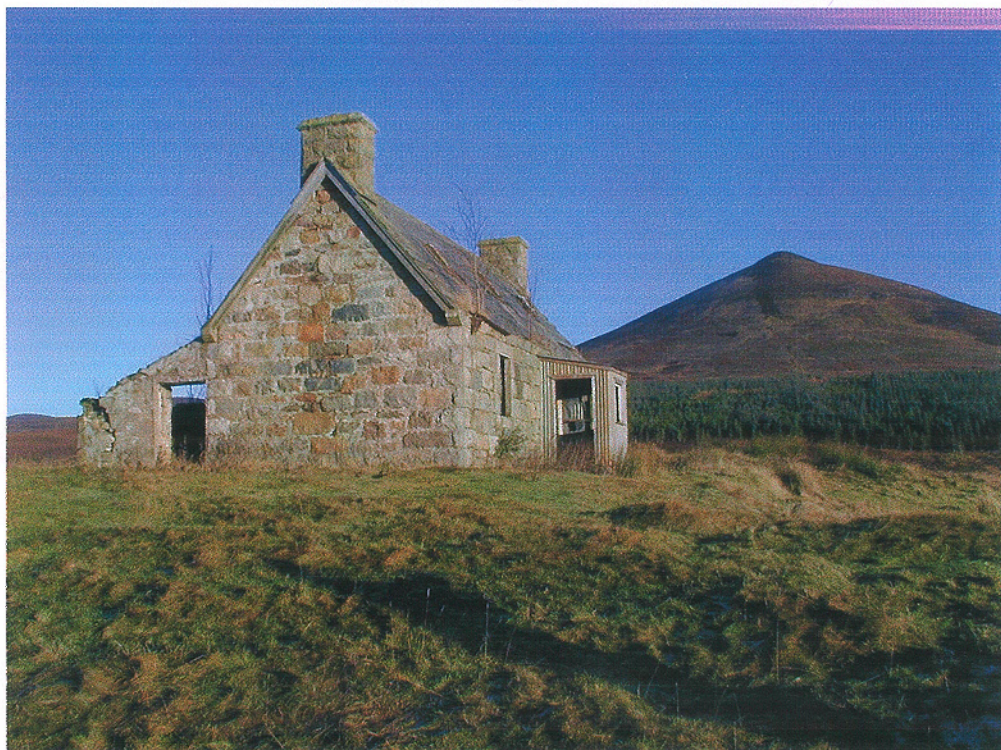
Plate 23. Feature 165. Derelict building at Upper Breac-achadh. (Gable end is 5m wide) GR 284855 911768
