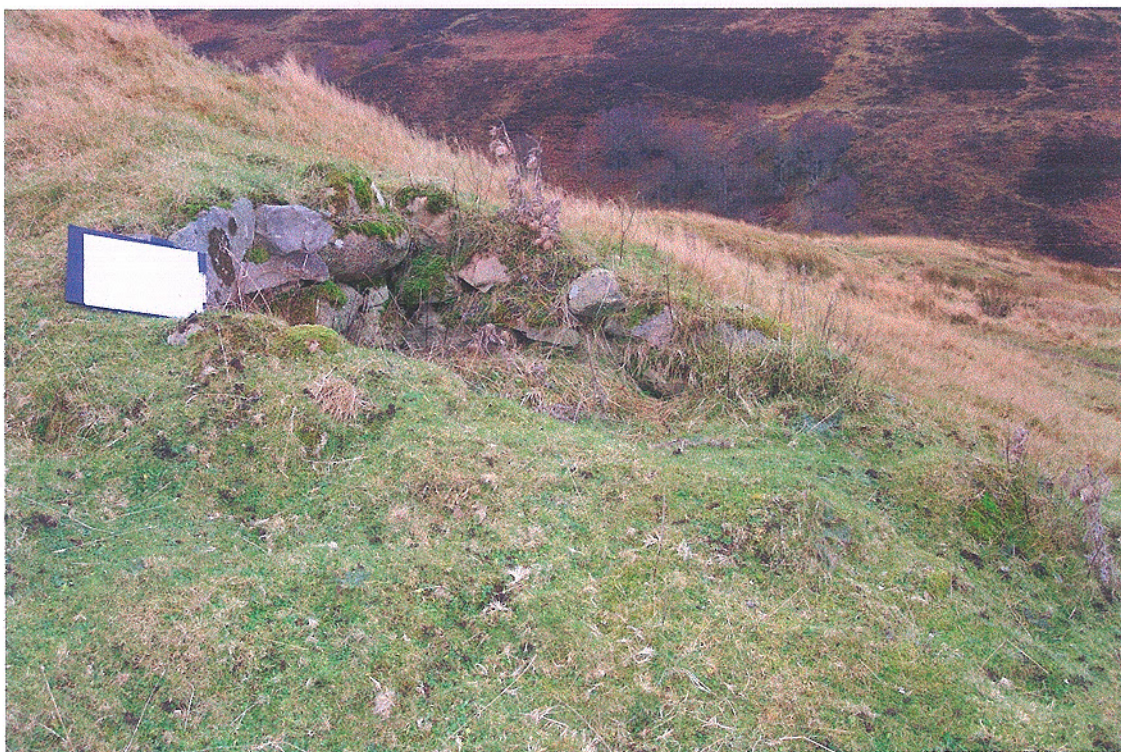
Plate 24. Feature 167. Small stone-lined platform recessed into slope at front of the derelict building of Feature 165 at Upper Breac-achadh. (Scale on top of structure is A4 paper) GR 284878 911736
